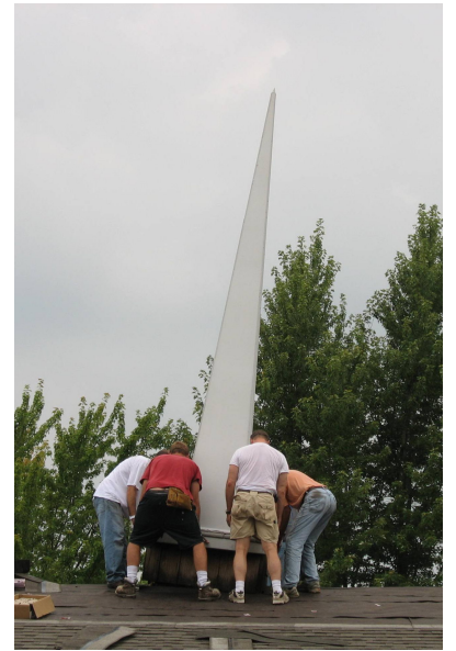
Step Two of the steeple removal
