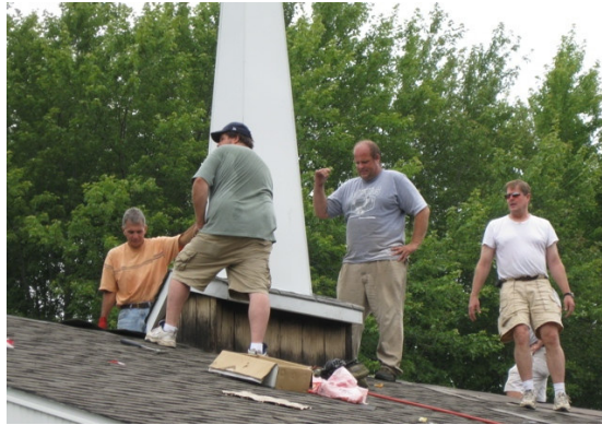
Step One of the steeple removal
